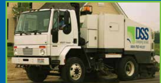
Construction Site/ Broom Sweeping
